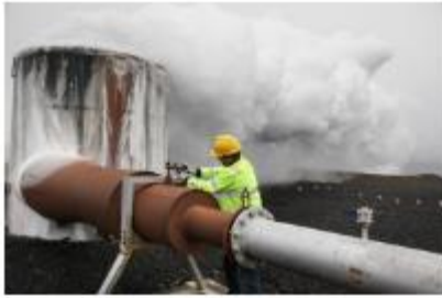
CarbFix project scientist Bergur Sigfusson checks a valve at a test well near the geothermal plant. (© AP Images)
