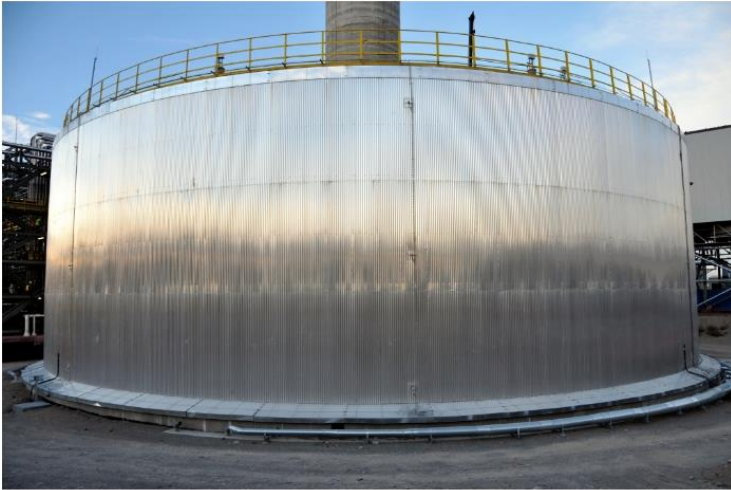
A huge tank at Crescent Dunes stores salt used to extend electricity storage capacity. (Courtesy photo)
