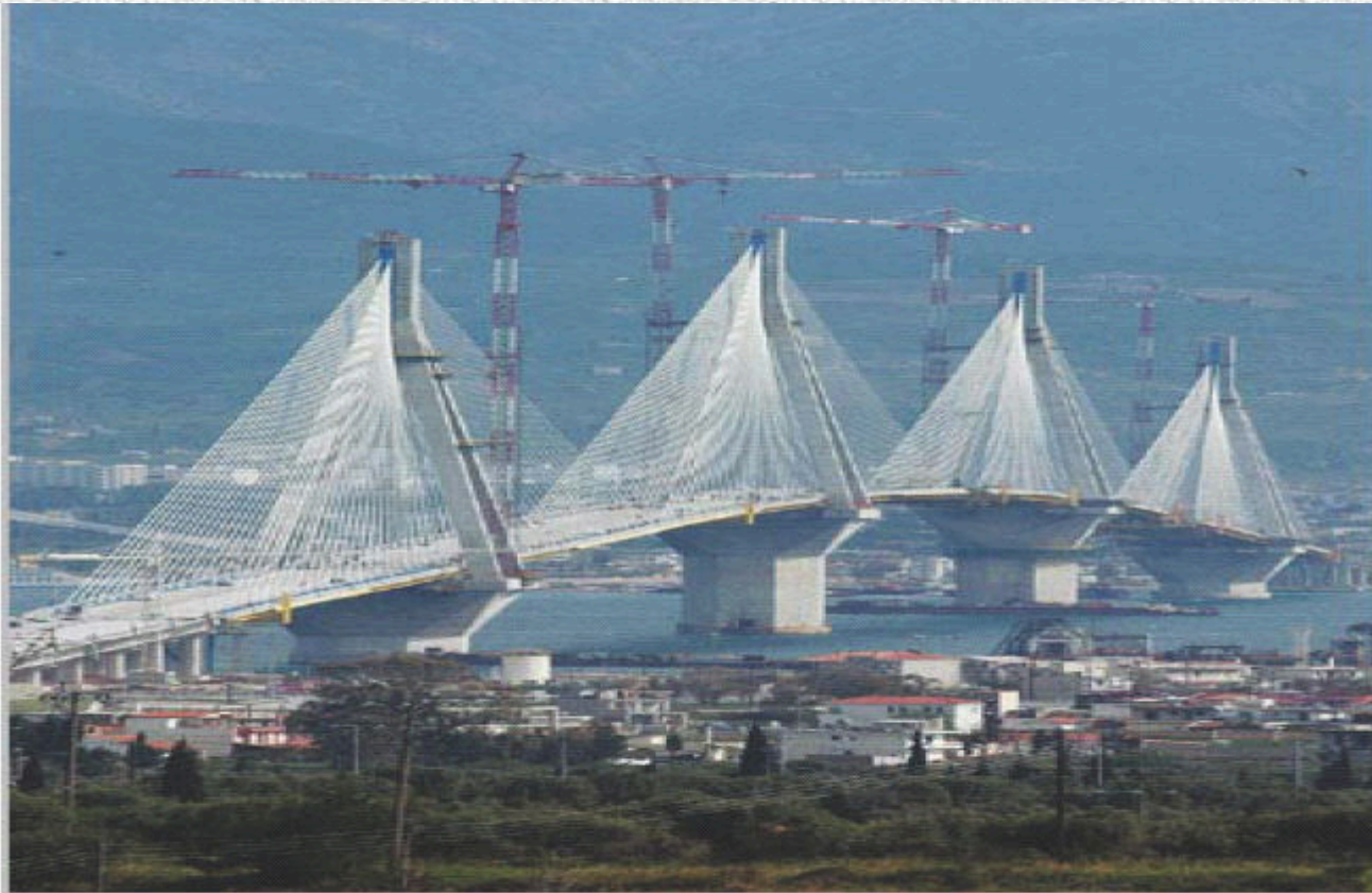
Rio-Antirio Bridge constructed with CEM III/A 42.5 cement (sea structure) and CEM II/B-M 32.5 (overland structure)
